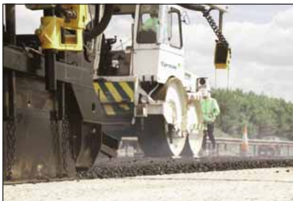
Asphalt being laid on the M1 Contract
