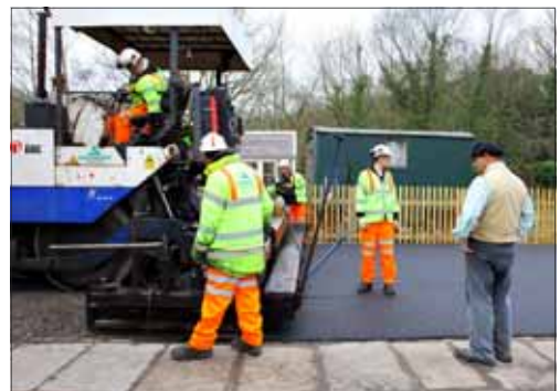
Victorian highway; modern technology
