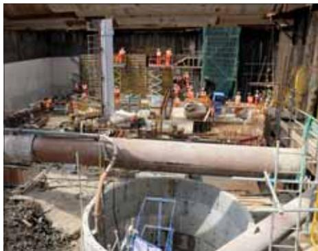
Excavation for TCR lift shaft down to the platforms
